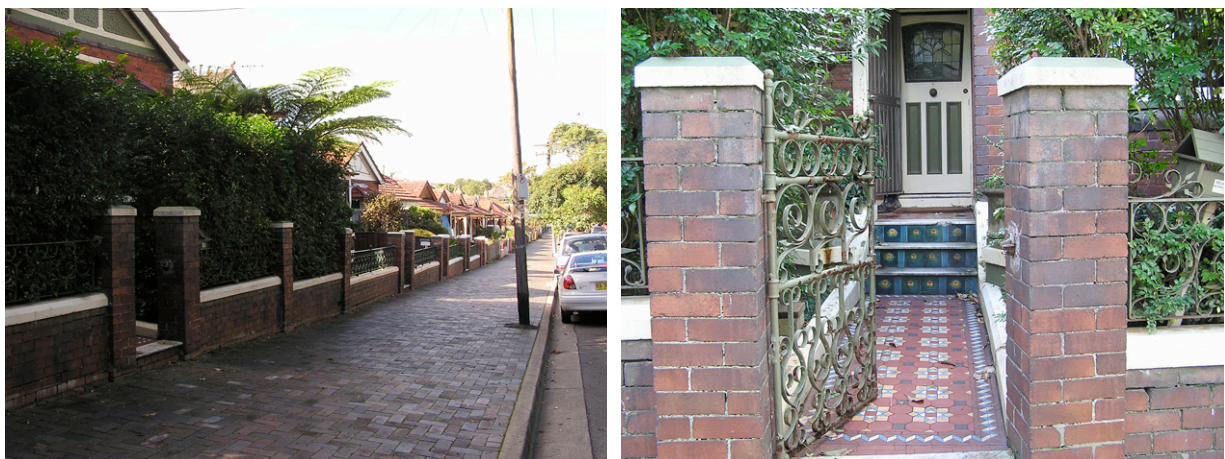
Figures 14.26 and 14.27. The later houses built in Victoria Road overlooking what is now the Marrickville Metro shopping centre demonstrate the fence style that became popular after the iron palisade. It consisted of a low brick wall (six to eight courses) with a worked iron ribbon panel fitted between two slim pillars with a matching gate. Note also the decorative tiles to the stair risers and the tessellated tile paving.
