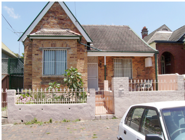
Figure 14.36. This house has been substantially altered through removal of render, replacement of windows and roof cladding and reconfiguration of the fence. The overall form remains relatively intact.
